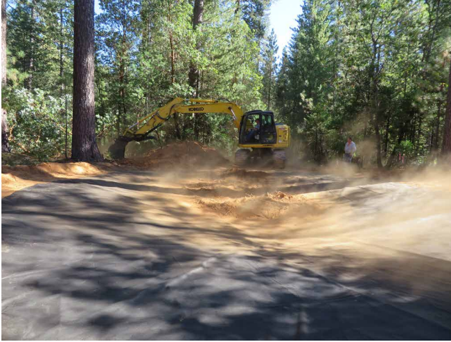
Filling trimmed and staked liners with 6 to 8 inches of soil.
